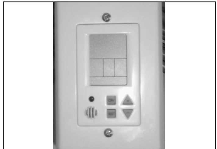
Figure 5 – Remote Thermostat Control
